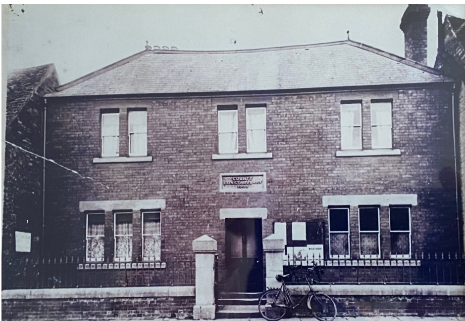
Cricklade Police Station as it looked in 1902, when first built and before the 1960s 'enhancements'
