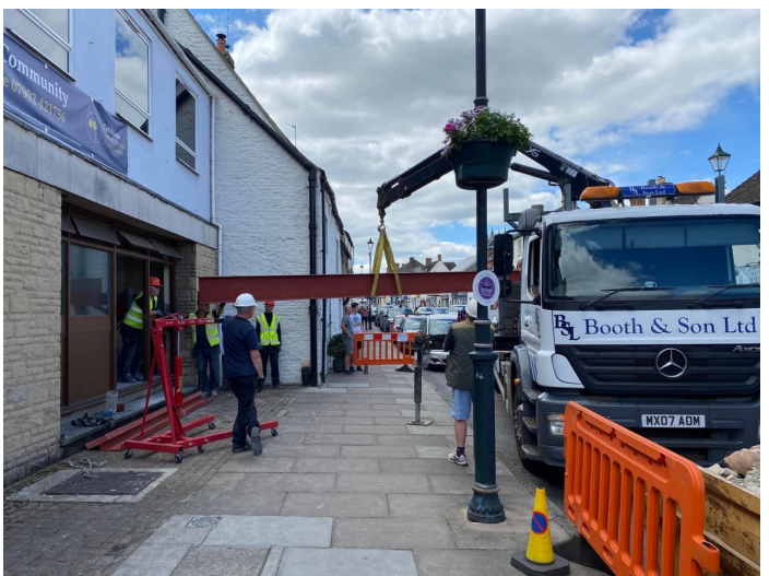
The RSJs (i.e. the "steels") being delivered - 13th June 2022
